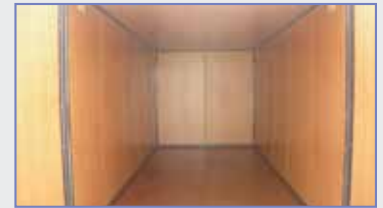
Retrofitted with laminated plywood floors and walls. Floor load 154 psf.
